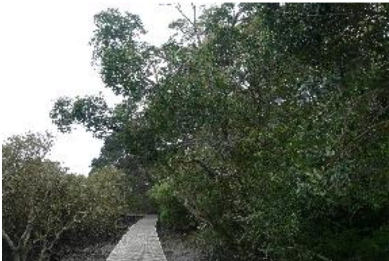
Weona Lemington Walkway completed 2017.
